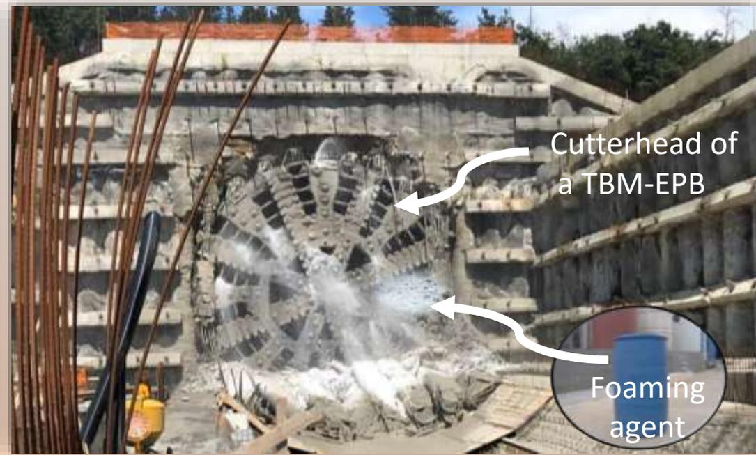
**Earth Pressure Balance - Tunnel Boring Machines (EPB-TBMs) functioning requires the use of additives, such as commercial foaming products (FA). FA are mixtures of various chemicals; most of them contain the anionic surfactant sodium lauryl ether sulphate (SLES)**
